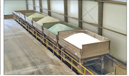
Five major product bins have a 16-ton capacity each from the new 15,000-ton building.
